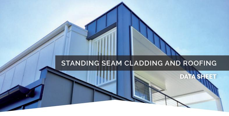
Offering a concealed fixing technology, Standing Seam can be applied to concave, curved, conical, flat and domed applications.
